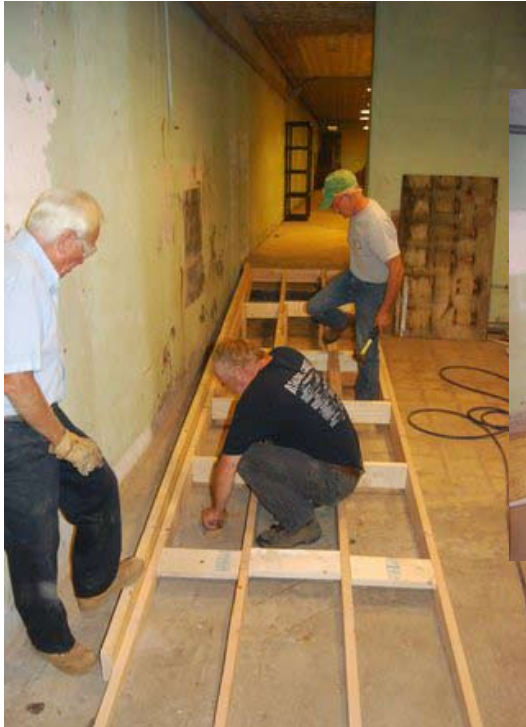
Working on a new handicap ramp
