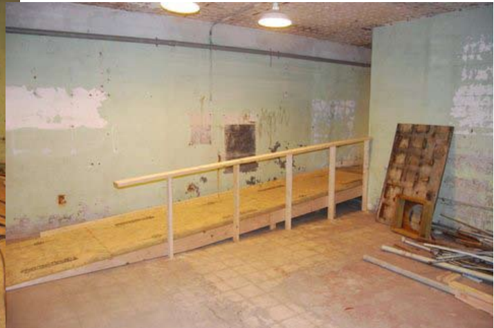
Working on a new handicap ramp
