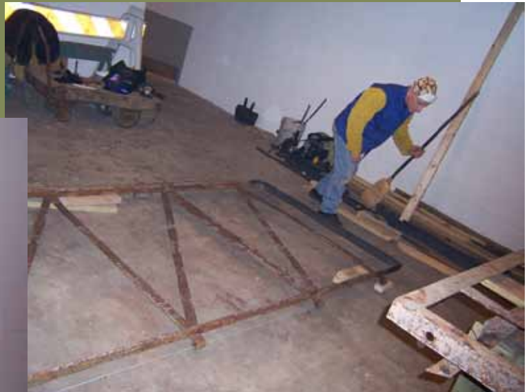
Working on the gates
