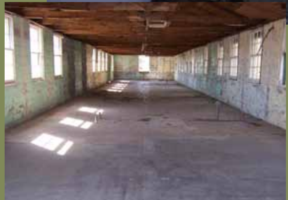
Restoration of Barracks T603
