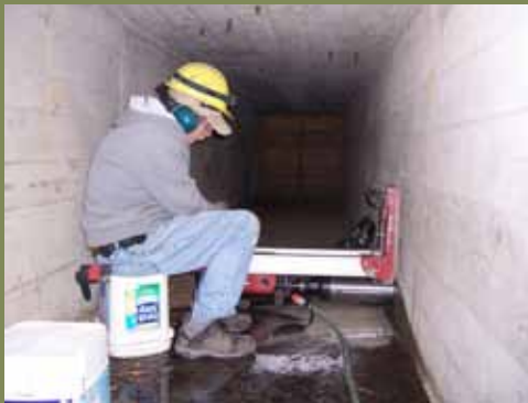
Boring holes for geothermal lines
