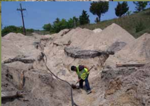
Digging wells and trenches for the Geothermal unit
