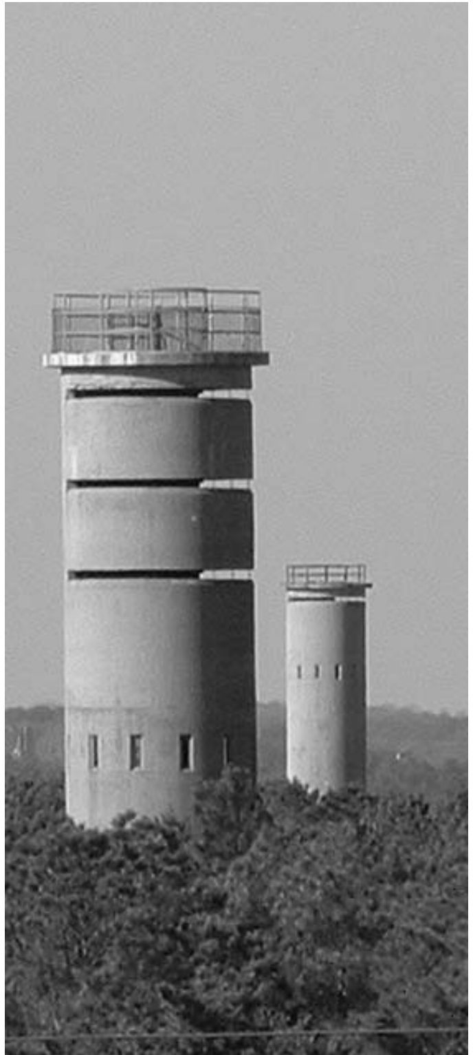
Fire Control Tower 7 (foreground) was a spotting station for the mines beneath the surface of the Delaware Bay. Fire Control Tower 12 (background) was the Harbor Defense Observation Post. The SCR-582 Radar Tower footings remain bolted to the very top of Tower 12.
