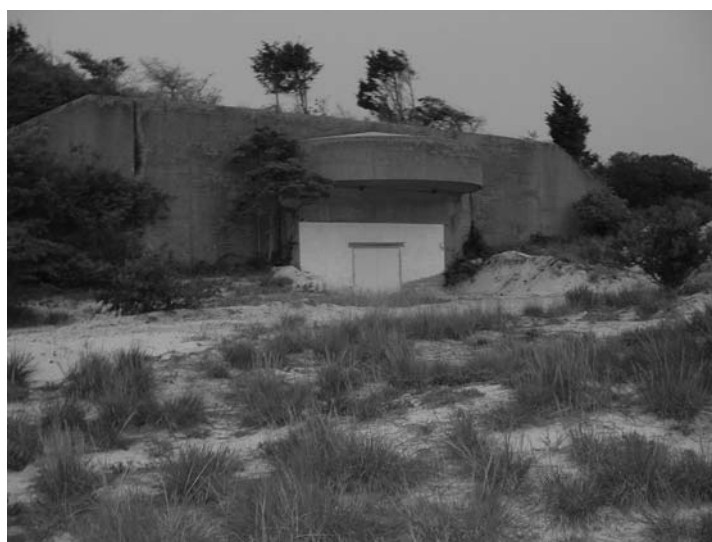
Battery 519's south gun block (above) will soon be home to a fully restored 12 inch artillery gun. The battery will be the centerpiece of the finished museum, the huge gun no doubt one of its major attractions. Its barrel will be colossal, reaching some 30 feet out of the building toward the sky. The gun is scheduled to be mounted in the summer of 2005.
